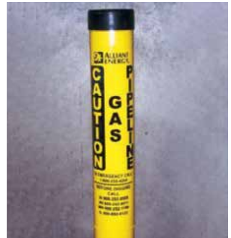
Alliant Energy Pipeline Makers – Found at road crossings, fence lines and street intersections. Markers do not indicate center of pipeline.
