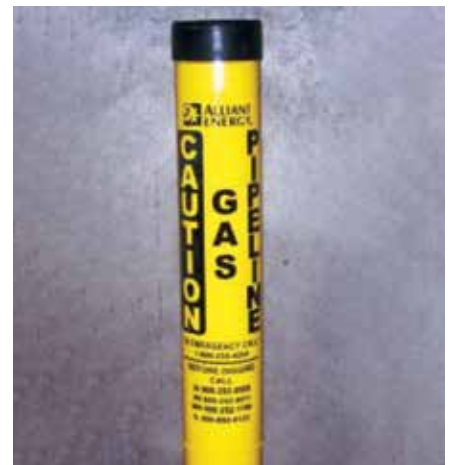
Alliant Energy Pipeline Markers – Found at road crossings, fence lines and street intersections. Markers do not indicate center of pipeline.
